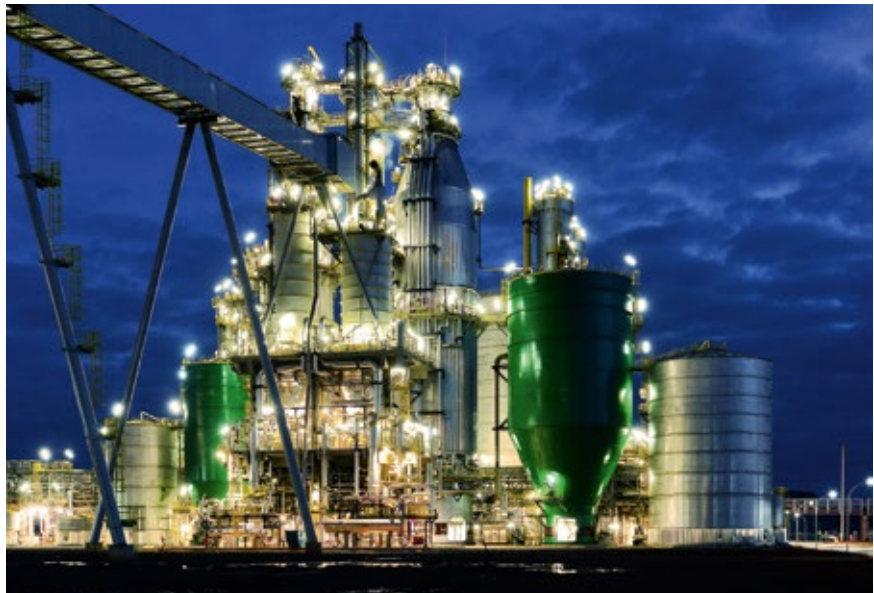
Pulp mill of an ANDRITZ customer in Brazil
